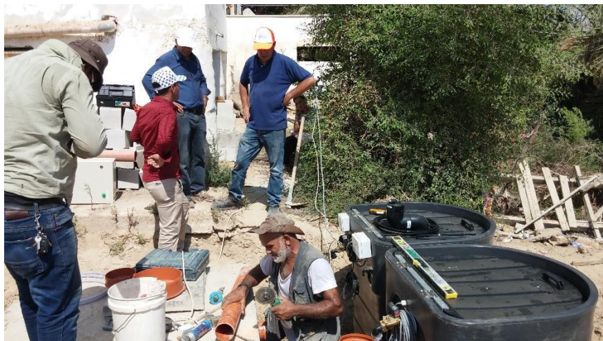
Picture 12 –Installation of Auja MBR System. September 29 th 2015
