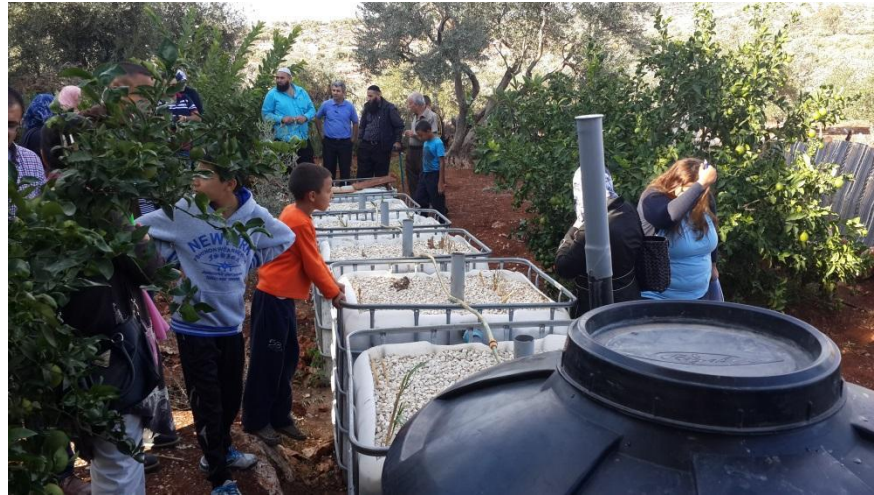
Picture 6 –Monitoring Deir El-Hatab Demonstration greywater treatment system
