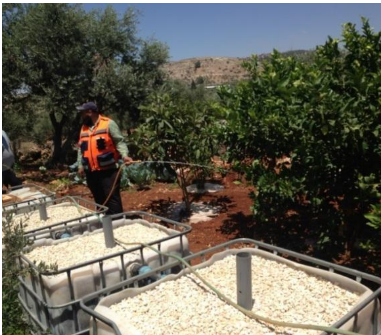
Picture 3 -Deir el Hatab household demonstration greywater treatment system
