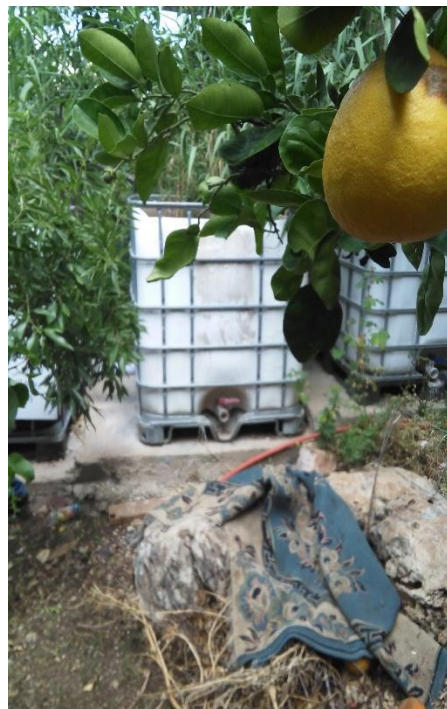
Picture 11 –Monitoring Zawata Demonstration greywater treatment system. Site visit May 20 th 2015.
