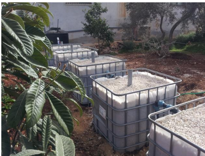
Picture 4 – Demonstration Greywater treatment system in Deir el Hatab.
