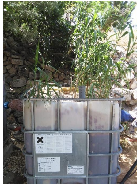
Picture 10 – Demonstration Greywater treatment system in Dar Salah. Site visit May 20 th 2015
