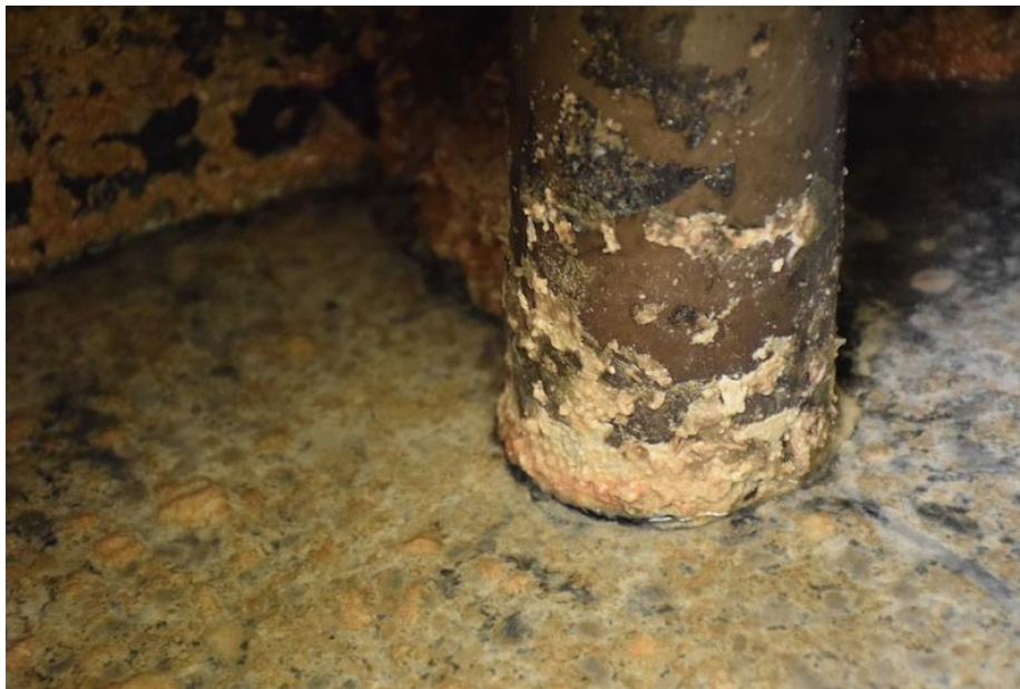
Figure 3: Surface crust and the siphon in the inflow collection tank. The siphon draws from about 30 cm below the surface. Photo credit: Antonia Bacigalupa Albaum
