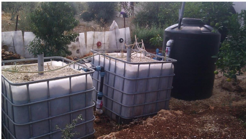
Figure 4: (right to left) Inflow collection tank and first 2 gravel treatment tanks of the CW system at Deir al-Hatab. Photo taken on the October 2014 CTWM monitoring trip.
