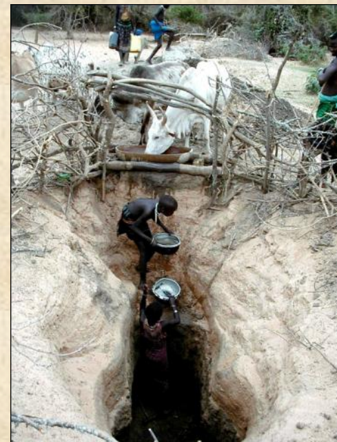
Shallow wells are dug into dry-creek loose sediments. Very low yields and poor safety setup
