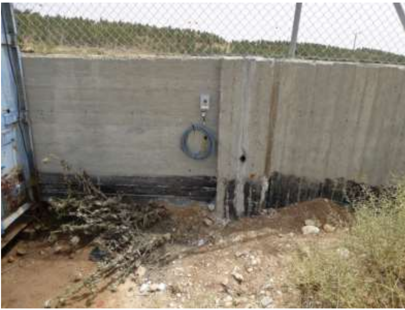
Figure 2: Storage system and transmission site located within the grounds of the WWT site to prevent vandalism
