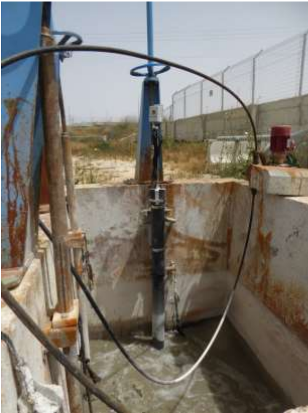
Figure 5: Water quality measurement station in the Hebron stream installed in a holding area at the collection site of the WWT facility.
