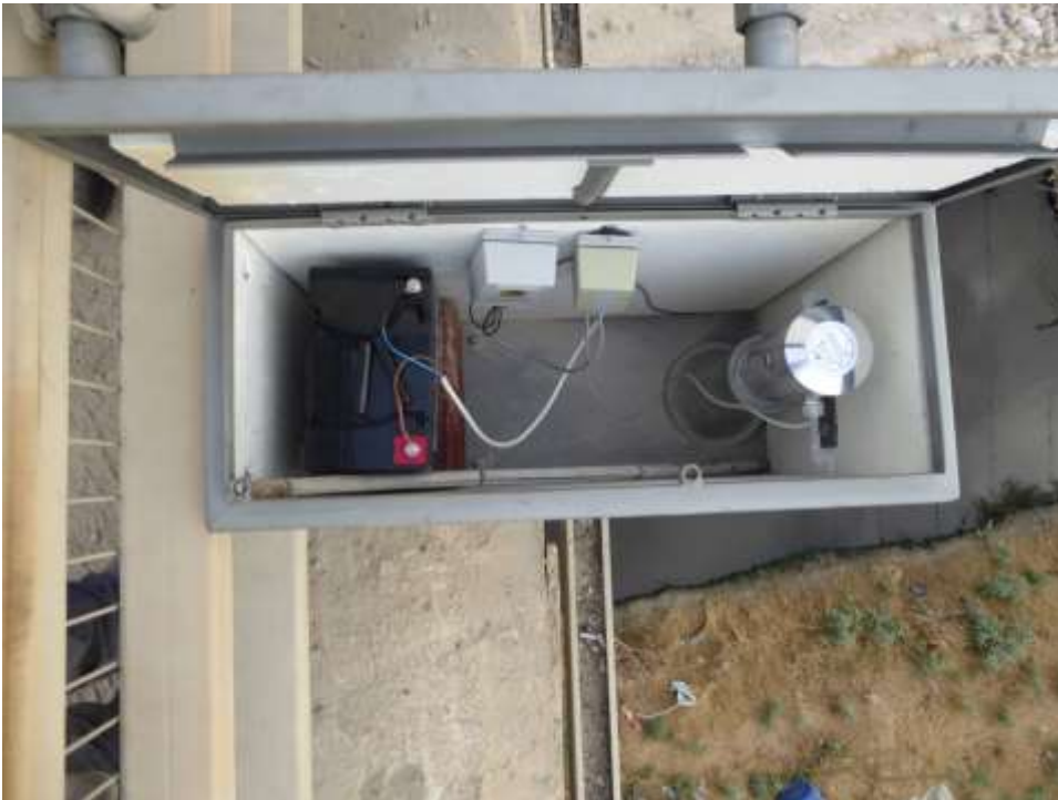
Figure 9: Instruments in the container padded with Styrofoam. The internal battery and battery supply energy for the system for about six months to a year.
