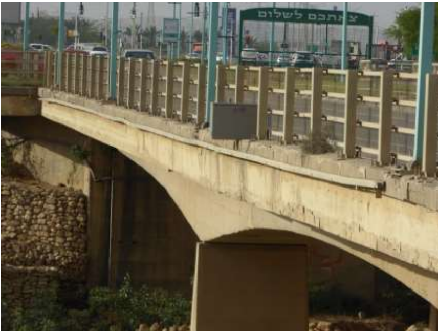
Figure 7: The radar station was installed on the bridge at the southern point of Beer Sheva to monitor water levels and flow rates in the Beersheba stream
