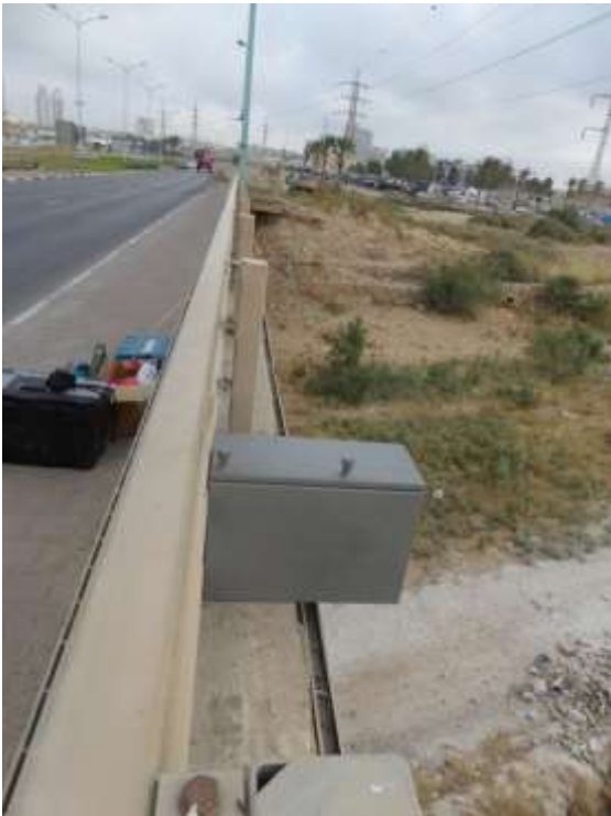
Figure 8: The container in which the instrumentation is located. The container is painted to blend with the environment, has special locks, the hinges are internal, and there are no external signs that there is an electronic system in it (such as a solar panel or antenna)
