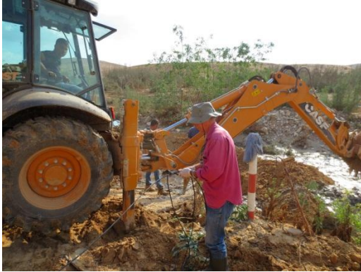
Installation process for a monitoring station
