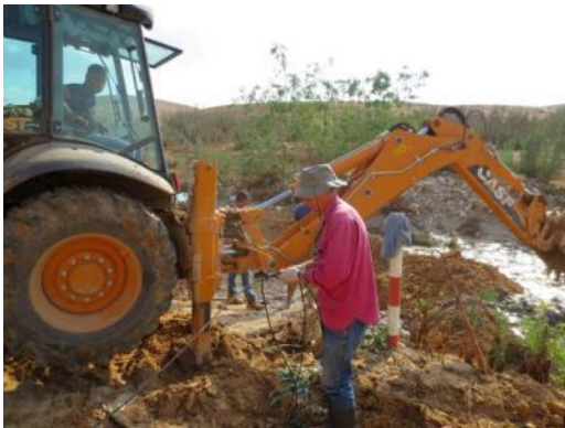
Installation process for a monitoring station
