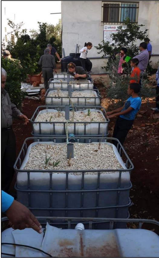
Image Credit: AIES Workshop participants tour an Arava Institute grey water treatment system at a family home in Nablus.
